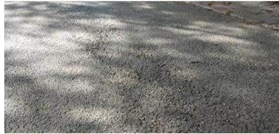
Gambar 4 Pelepasan Butir (*weathering and raveling*)
