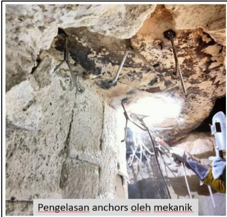
Gambar 6. Pengelasan anchor didalam cyclone 4A
