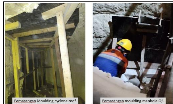
Gambar 8. Pemasangan moulding didalam cyclone 4A
